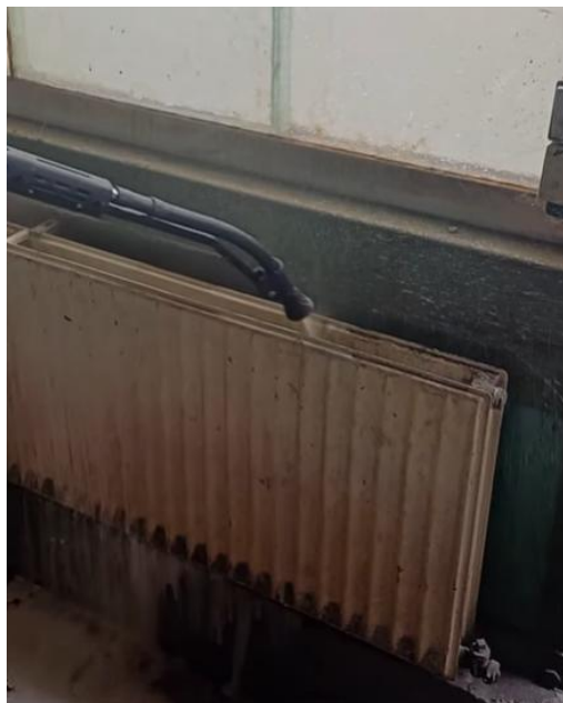
Flat radiator - before (with cleaning between the panels)
